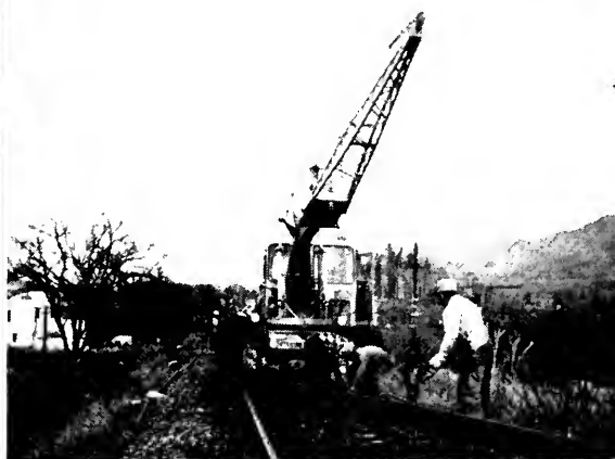
LAYING STANDARD RAIL
